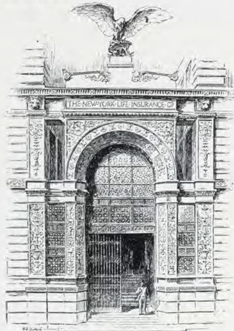
Entrance, New York Life Insurance Building, built in 1888-89, and razed.
