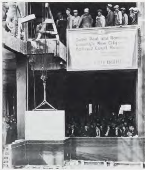
Laying of the cornerstone for the new city hall/courthouse in 1931.
