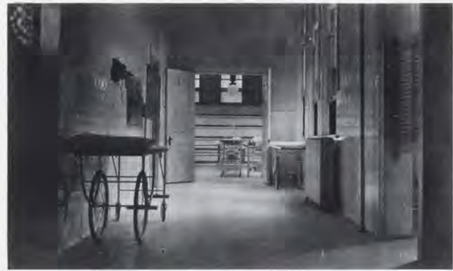
Corridor leading to Emergency.
