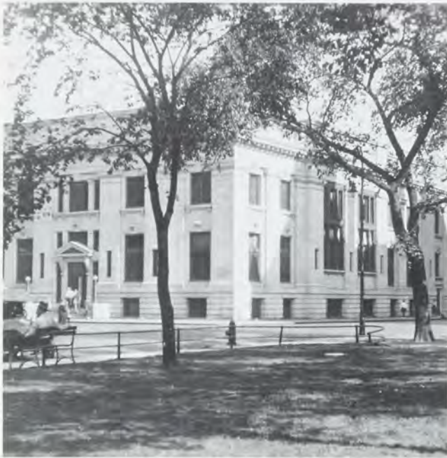
The company's second home office building, above, opened in 1909 at the corner of Fifth and Washington streets, a site once owned by Alexander Wilkin. In 1961 the company's headquarters were completely rebuilt on the same site. Both are viewed here from Rice Park.
