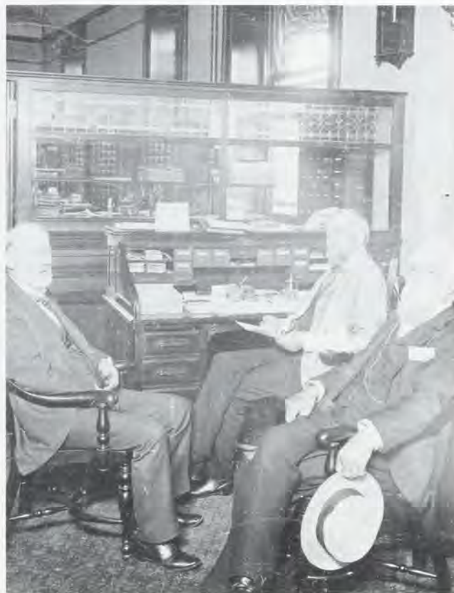
Amherst H. Wilder, left, and Captain Peter Berkey, right, company directors, with Charles H. Bigelow, president, in the company's first home office building in 1894. This was the building with a steam gauge and speaking tubes.
