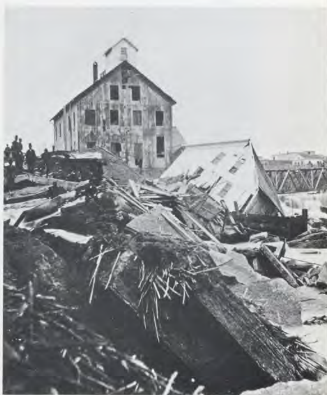
The "tunnel disaster" — St. Anthony Falls after an attempt to build a tunnel underneath failed.
