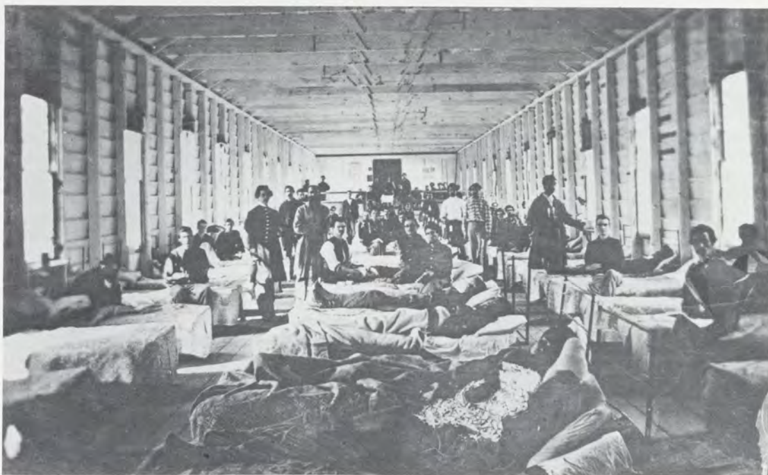
A Civil War hospital, similar to the base hospital of today.
