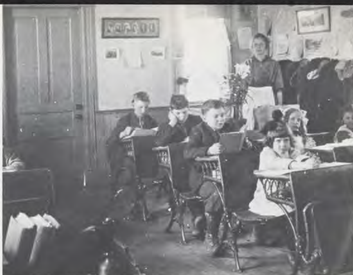
First classroom: Wooden desks with fancy iron scrollwork and a row of hooks on the wall for coats. The author stands beside them.
