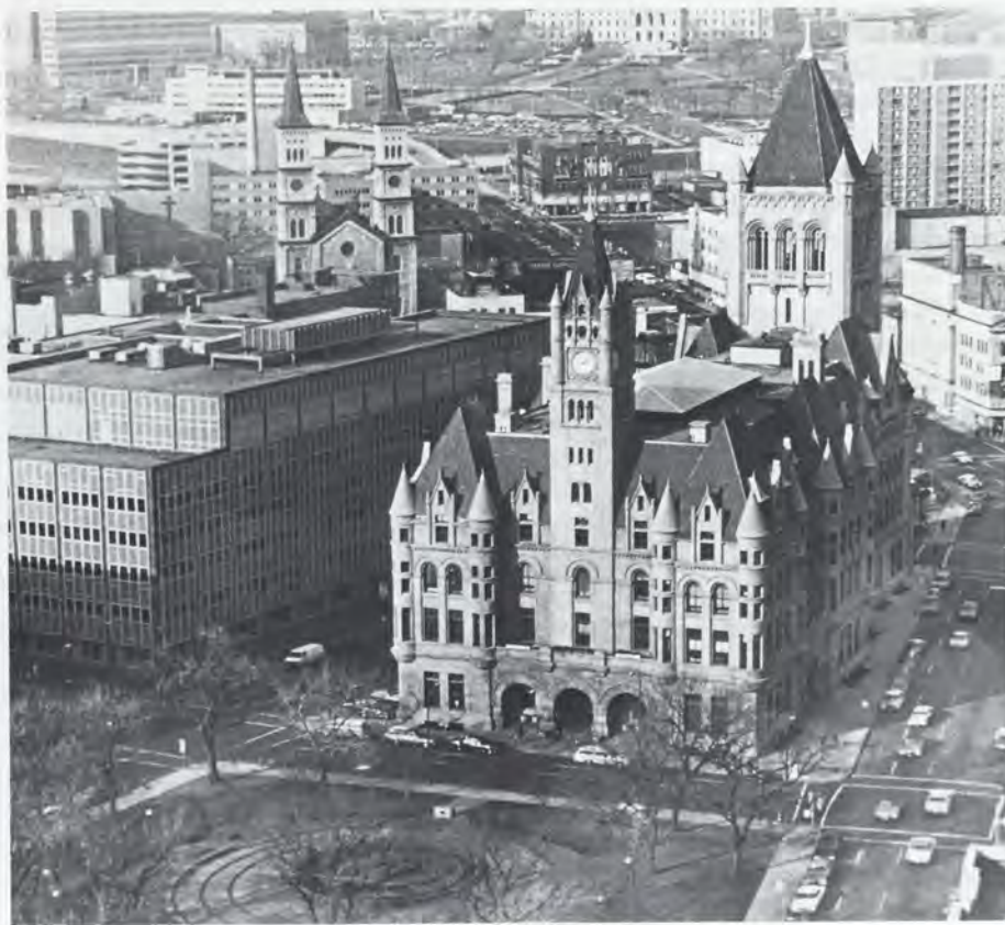
Landmark Center, the former Old Federal Courts Building, now restored as a cultural center with the help of The Saint Paul Foundation.
