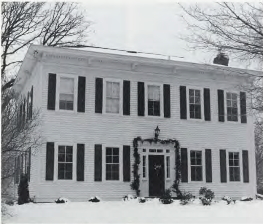
The Davern house at 1173 Davern Street in 1990.
