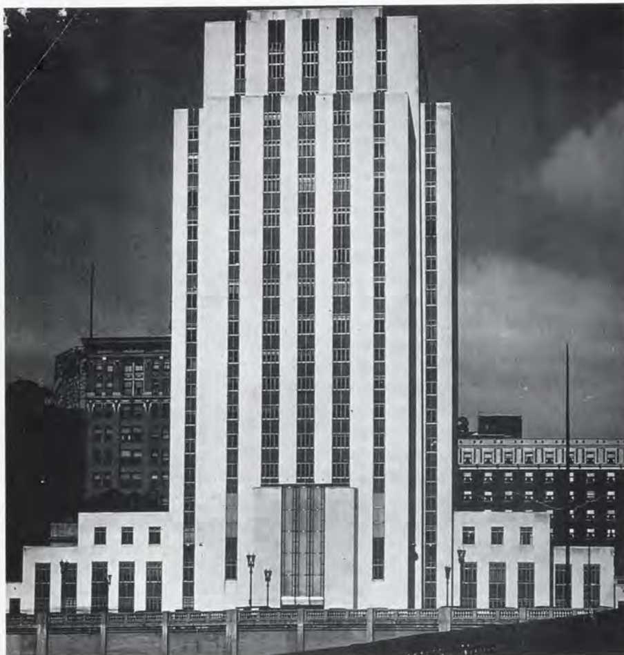
The city hall and county courthouse soon after its completion in the early 1930s. Unless otherwise noted, this and other Hedrich Blessing photographs of the building's interior have been reprinted from an article published in American Architect in the mid-1930s.
