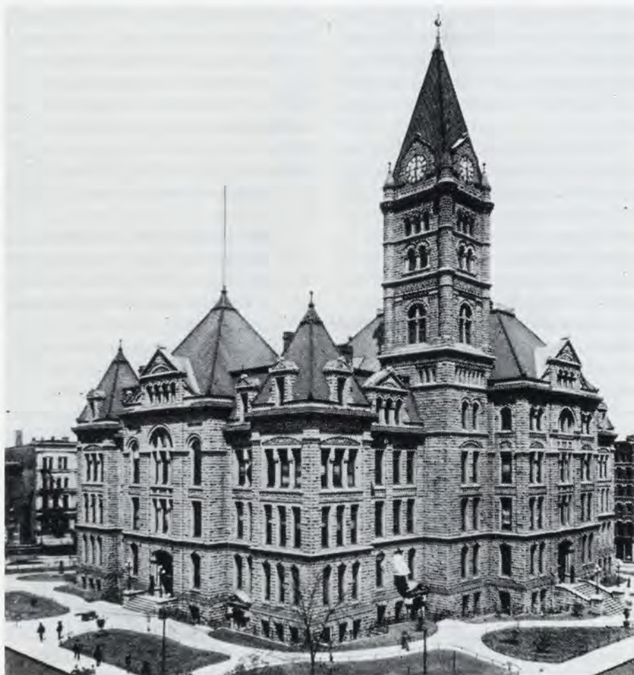
The castle-like 1880s city hall-country courthouse around 1910. C. P. Gibson photo, Minnesota Historical Society.
