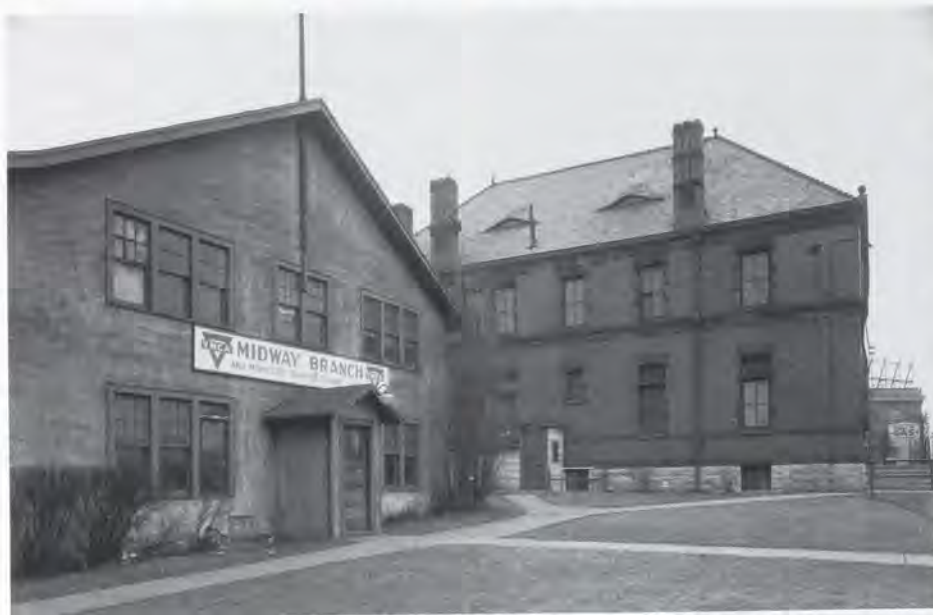
The YMCA's old building at Prior and University Avenues. The $6,000 building opened its doors in the Fall of 1921. Kenneth M. Wright photo from the Midway Chamber of Commerce.
