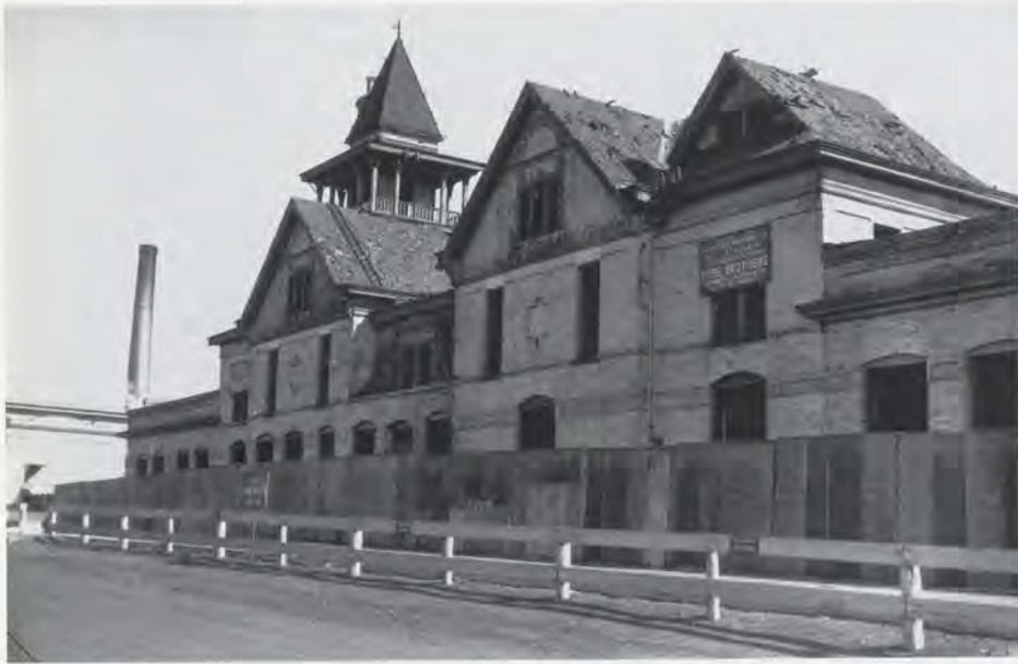
Norman W. Kittson's stables at University and Snelling before their demolition in 1942. Minnesota Historical Society photo.
