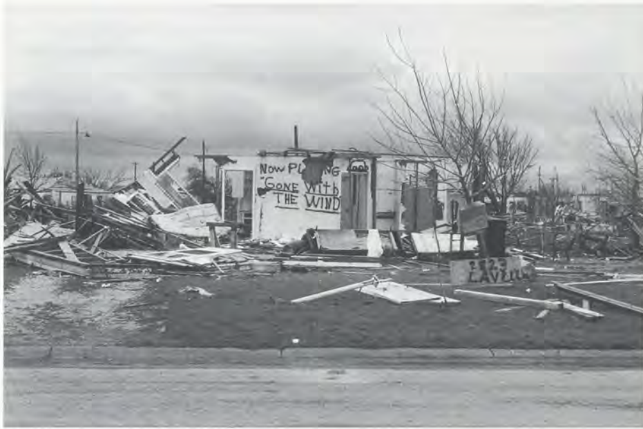
Truly gone with the wind. Damage from the 1979 tornado at Wichita Falls, Texas.
