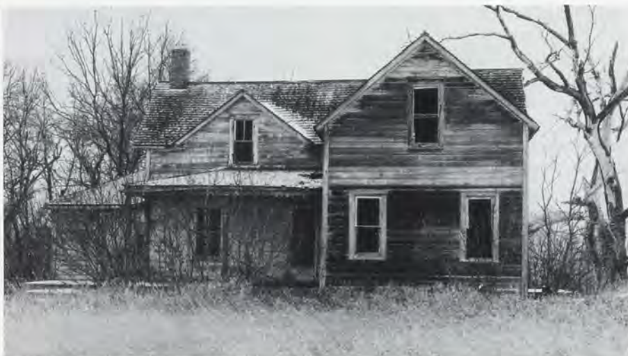
A classic Minnesota L-house. The arrangement of the rooms, with the kitchen porch opening to east and south where the barnyard lies and the formal front of the house facing the road to the north, is typical of these farmhouses, Gabler writes. Photograph from the book.
