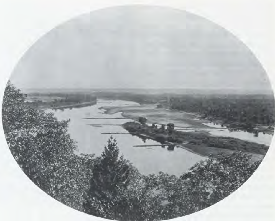
Life on the Mississippi: "The military engineers of the Commission have taken upon their shoulders the job of making the Mississippi over again—a job transcended in size by only the original job of creating it. They are building wing dams here and there, to deflect the current; and dikes to confine it in narrower bounds; and other dikes to make it stay there; and for unnumbered miles along the Mississippi, they are felling the timber-front for fifty yards back, with the purpose of shaving the bank down to low-water mark . . . and ballasting it with stones . . . One who knows the Mississippi will promptly aver . . . that ten thousand River Commissions, with the mines of the world at their back, cannot tame that lawless stream . . ." This is Bosse's photograph of wing dams at Pine Bend.
