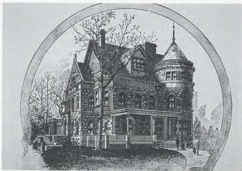
The house at 476 Summit Avenue that Chauncey W. Griggs built in 1883. Designed by Clarence H. Johnston, the brownstone structure cost $30,000. Minnesota Historical Society photo.
