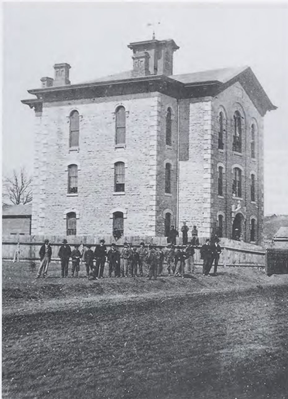
Franklin School at Broadway and Tenth Street under construction in 1865. A portion of Flanagan's taxes went to pay for it.
