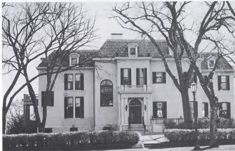
The Maurice and Matilda Rice Auerbach house at 400 Summit as it looked in 1882, in this photo from the Minnesota Historical Society, and the same house as it looks today. Lucius and Jessie Ordway moved here around 1918, perhaps because the house had an elevator. Later they remodeled it extensively.
