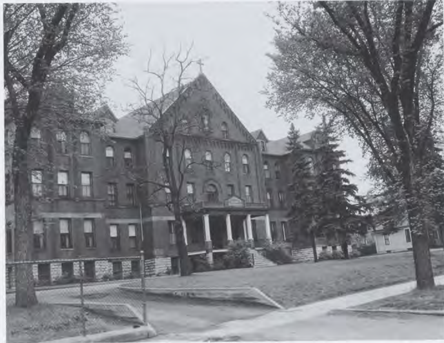
St. Joseph's Catholic Orphan Home at 1458 Randolph Avenue, St. Paul, as it looked in 1960, two years before it was torn down. St. Paul Dispatch-Pioneer Press photo from the Minnesota Historical Society collections.
