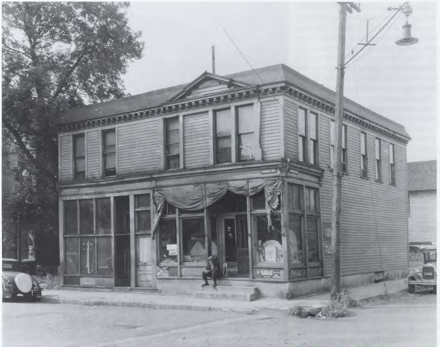
David Talbert's house at 553 Sibley. Talbert was a cook and caterer. He arrived in St. Paul in 1850 and is said to have helped slaves, who came to St. Paul with their Southern owners, escape to freedom.
