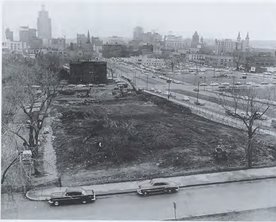
Nothing but vacant lots. This is Central Park Place West after it was cleared in 1958. The Macey, the Blood mansion and all the others are gone forever.
