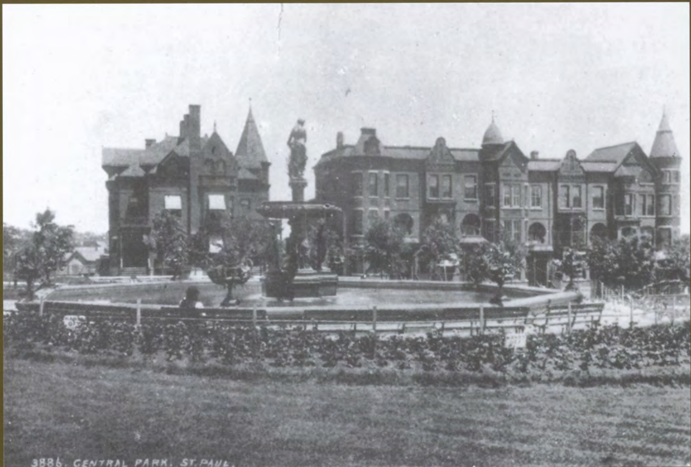
3886. CENTRAL PARK. ST. PAUL. The James Humphrey house on the left, the Gustave Schurmeier rowhouses on the right. See article, "The Life and Death of Central Park," beginning on page 4.
