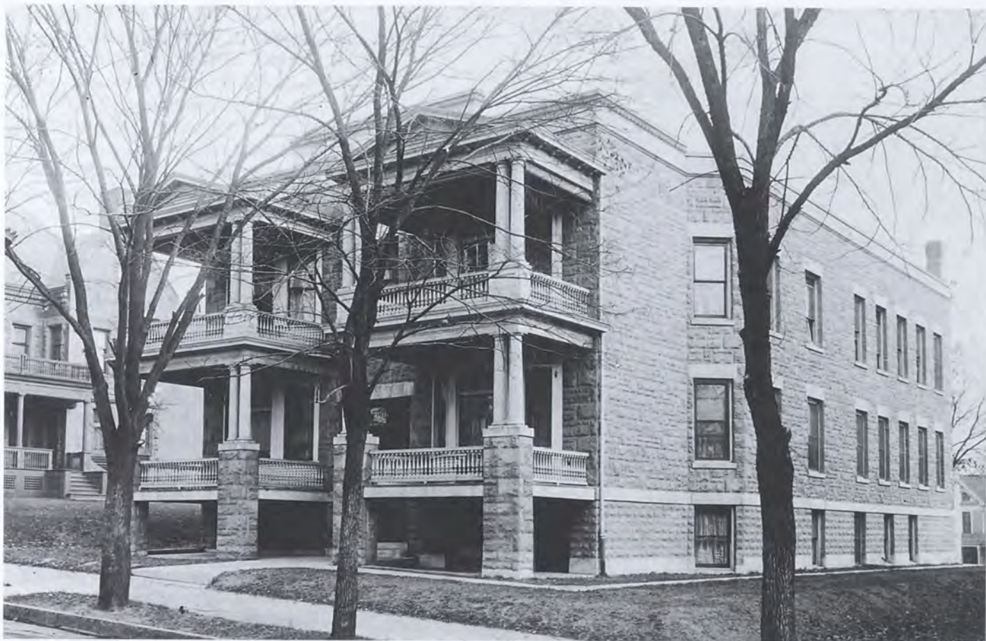
The Hurd Apartments at 638 Central Park Place, ca. 1910.
