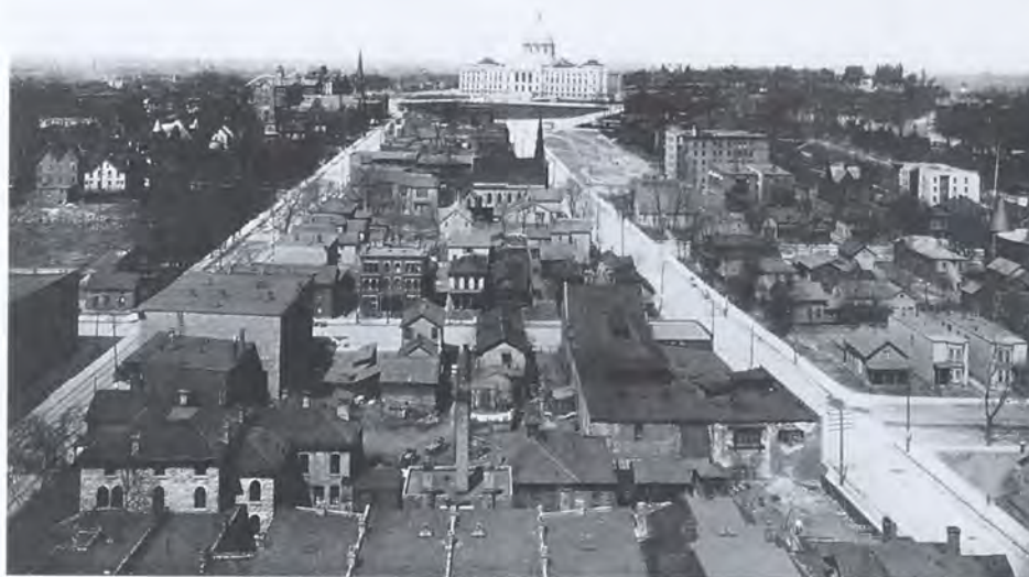
The "screen of ugliness" in 1930. At center right near the open space is the Macey; the white apartment building at the far right is the Brewster.
