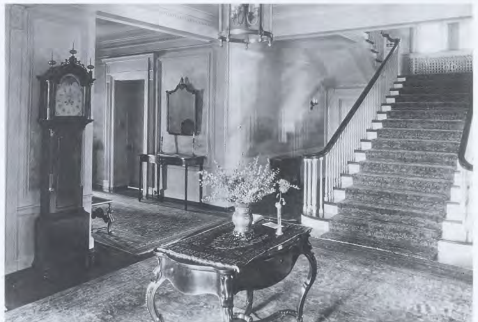
The mansion's first floor with its ten-foot-high center hallway and double switch-back stairway. Doorways on either side led to the servants' area. The depth of the concrete and hollow tile walls can be seen in the doorway at left. The grandfather clock, now in the possession of Oliver Crosby's great-grandson, came to America with the Crosby family before the American Revolution. A chest-high steel safe was located under the stairs. Photograph from the Minnesota Historical Society.
