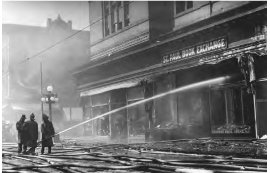
This newspaper photograph captures the destruction that the April 27, 1915, fire caused to Market House, which was then the home of the St. Paul Public Library. Photo courtesy of the Minnesota Historical Society.
