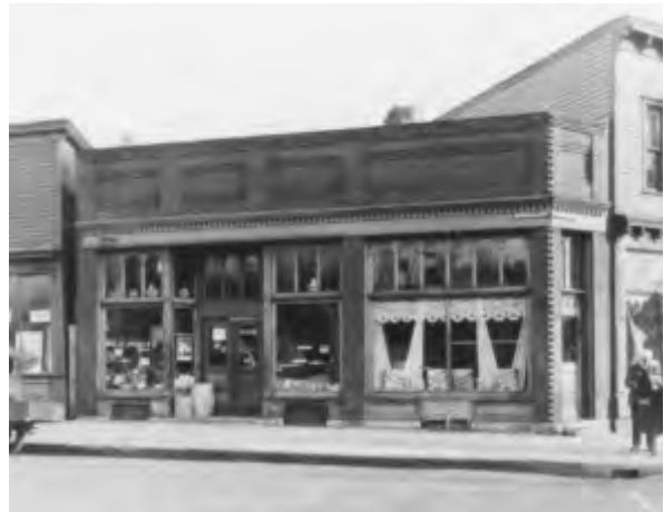
532 Decatur, built 1884 (same building as 534).
