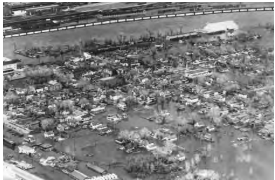
The West Side of St. Paul along the Mississippi River, including the Flats (bottom), during the March 1952 flood. St. Paul Dispatch photo. Photo courtesy of the Minnesota Historical Society.
