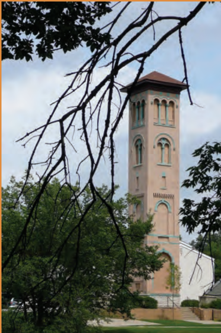
Torre de San Miguel (Tower of St. Michael) is a major landmark on St. Paul's West Side and a powerful emblem for Minnesota's first urban barrio. For more on the history of Mexican-Americans in this neighborhood and Minnesota, see page 20. Photo by Lelia R. Albert.
