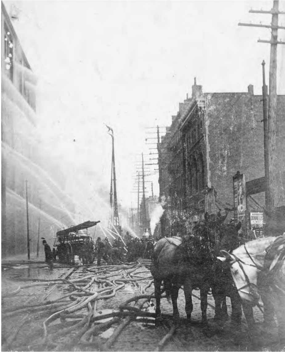
This photo of a St. Paul fire in 1900 illustrates how firemen usually fought industrial fires at that time. The firefighters are positioned close to the burning building, which was similar in height to the McCormick building that collapsed in the Midway fire. As part of the procedure for setting up to fight a fire, the horses that pulled the fire apparatus were released and secured at a distance for their protection. These firefighters are concentrating the water from their hoses on one area of the fire. Photo courtesy of the Minnesota Historical Society.
