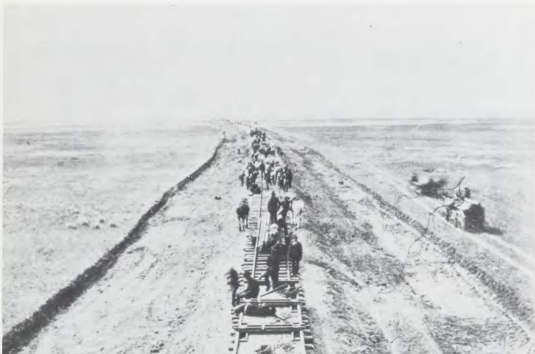
Laying track across the western prairie.
