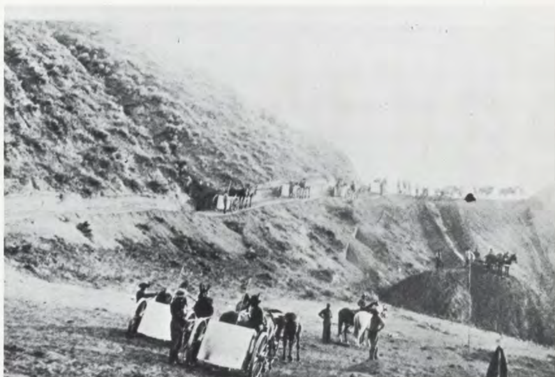
By 1882, grading was just being completed on the Great Northern line between Minot, North Dakota and Great Falls, Montana.
