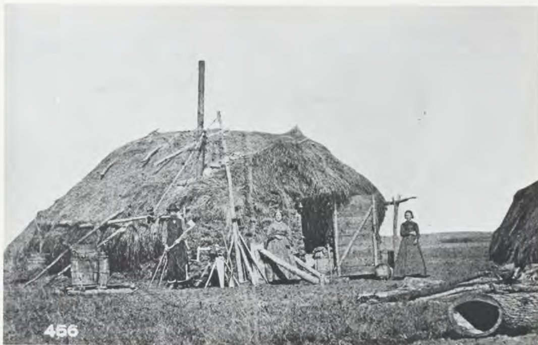
The soddy: its weaknesses were evident during heavy rainstorms.
