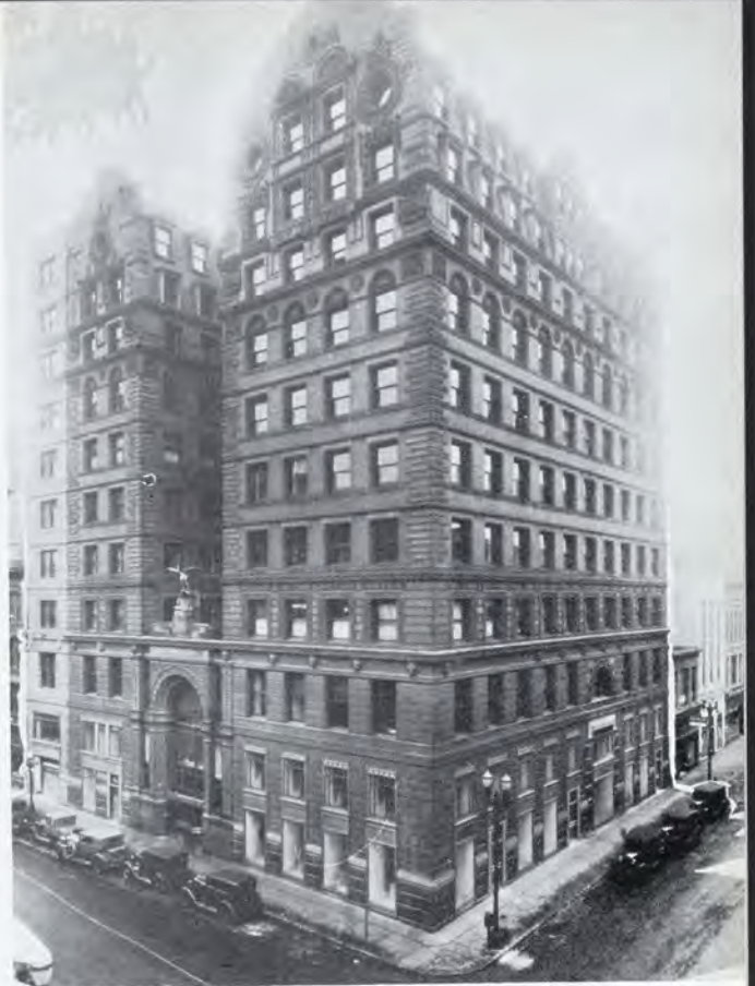
The New York Building shows a distinctly "Hanseatic" or northern German influence in design.
