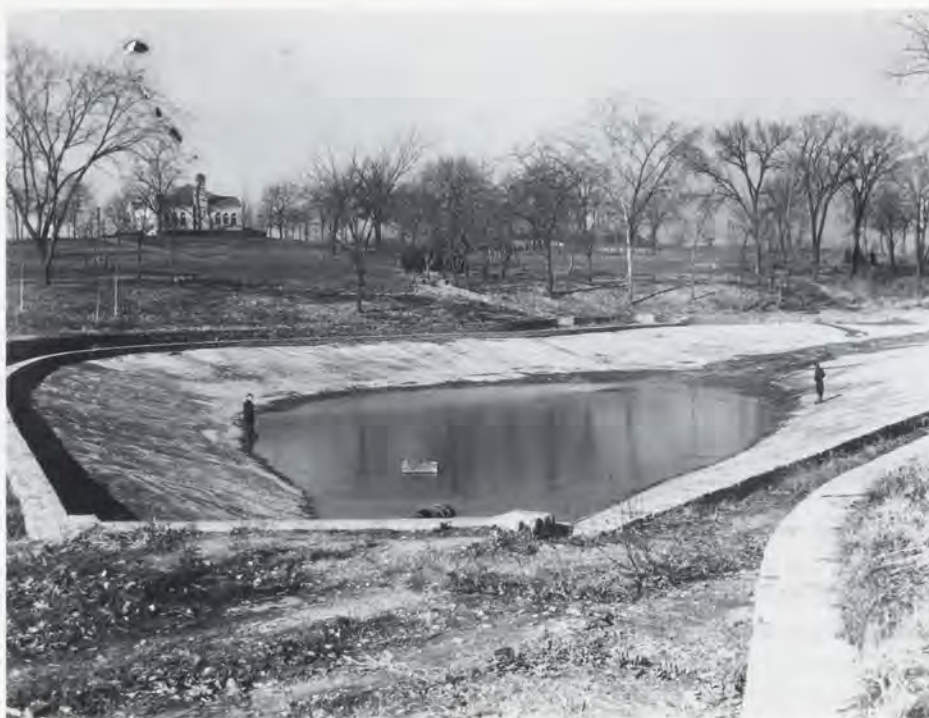
The Highland Park swimming pool, with the hazardous sloping sides. With WPA help, the pool was torn out and rebuilt.
