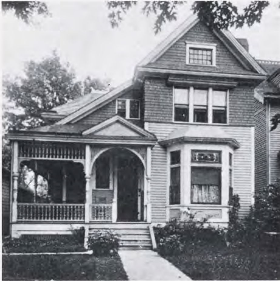
W. T. Francis' home at 606 St. Anthony Avenue.
