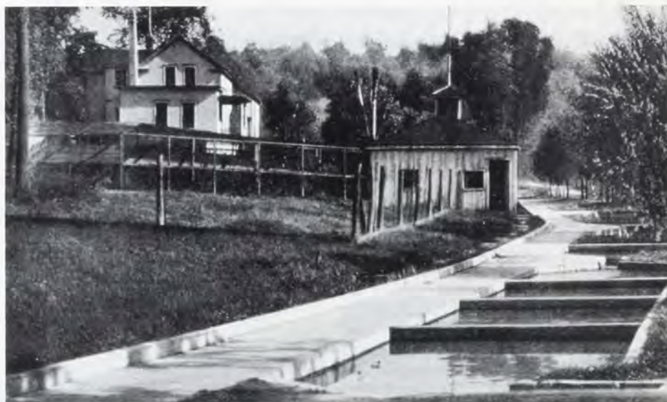
"Raceways" on the right, the superintendent's house on the left.
