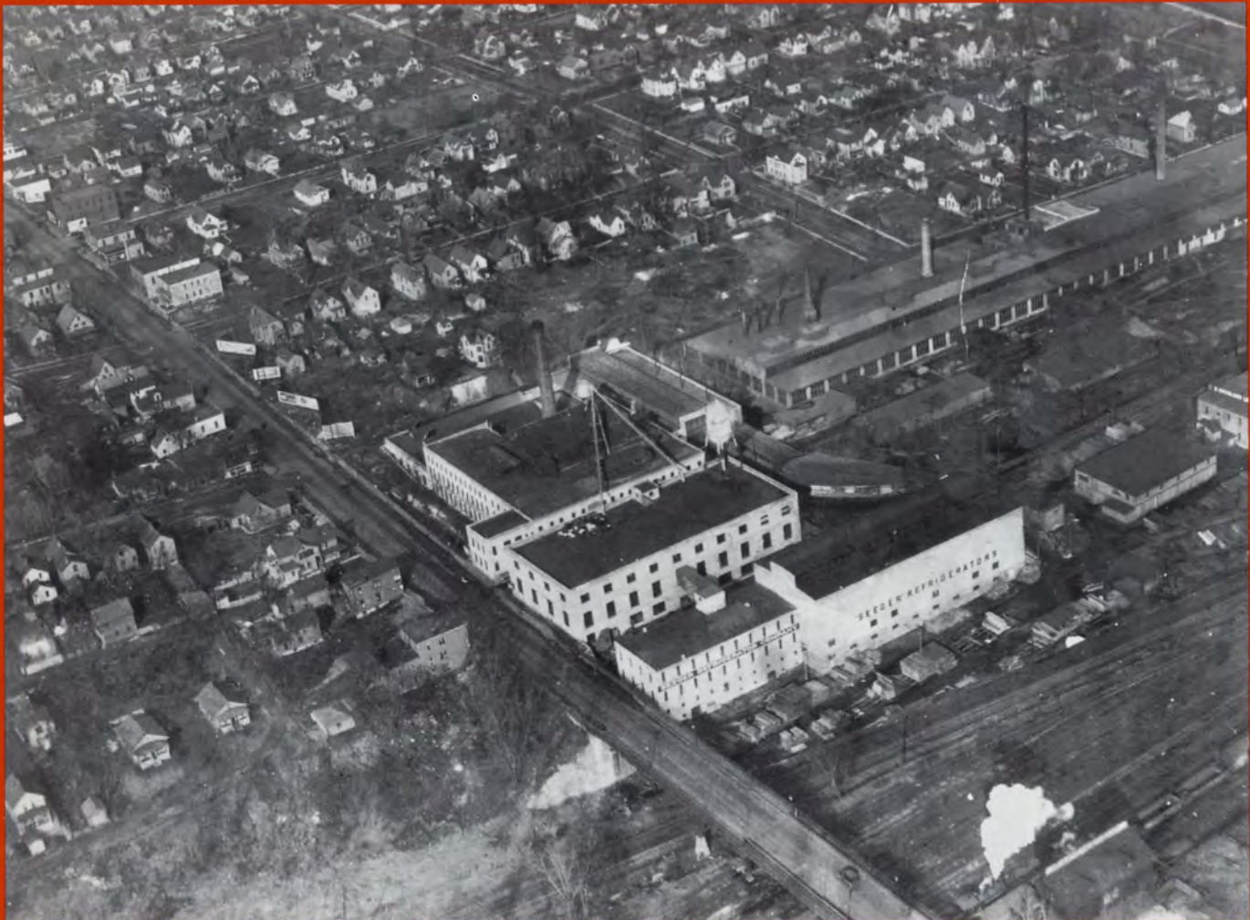
A view of the Seeger Company's Arcade Street factory, ca. 1930. The last building remaining at the company's site was razed in April, 1995. See article beginning on page 4. Minnesota Historical Society photo.
