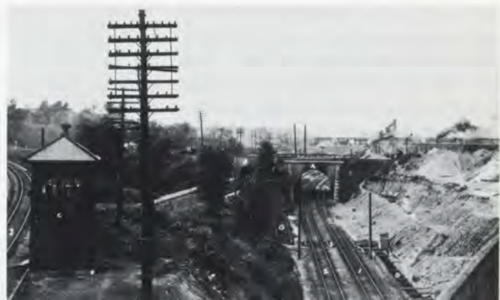
The junction in 1926. These views taken in September, 1926, show the Westminster Street tunnel beneath the east leg of the Chicago, St. Paul, Minneapolis & Omaha wye, and the tracks looking west from the Westminster Street bridge. Both photographs are from the Northern Pacific Railway Company records at the Minnesota Historical Society.
