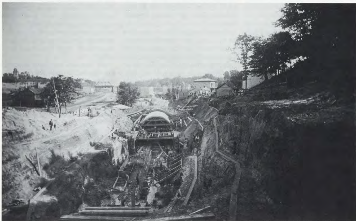
Westminster Junction tunnel, photographed on September 14, 1885. The junction, by the early 1920s one of the busiest in the Twin Cities, lies about one city block northwest of the Lafayette Road bridge. Two of its tunnels can be seen from the bridge. This view is looking toward the south. Photo courtesy of the National Railway Historical Society, North Star Chapter.
