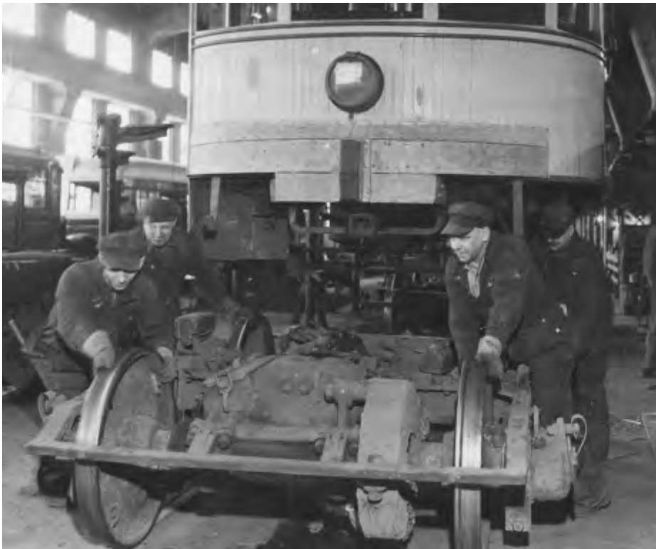
Workers at the Snelling Shops. An unidentified repair crew at the Snelling Shops removes the front truck and traction motor assembly from beneath a streetcar. Can anyone identify these men? St. Paul Dispatch and Pioneer Press photo, April 21, 1943. Minnesota Transportation Museum Collection.
