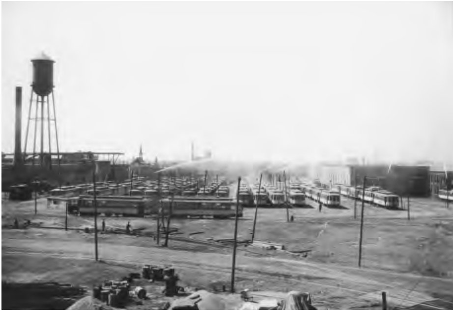
Snelling Shops. The shops, photographed circa 1925–1927, occupied approximately forty acres of land at the intersection of Snelling and University Avenues. They were the main shops for the entire TCRT system and were recognized as one of the finest maintenance and repair facilities in the electric railway industry. This view taken from the Montgomery Ward Department Store looks west toward Snelling. The Snelling car barn is on the right, paralleling University Avenue. The heavy repair shops appear on the far left and a large streetcar storage yard is in the middle. Workers are testing the fire protection system. Minnesota Transportation Museum Collection.
