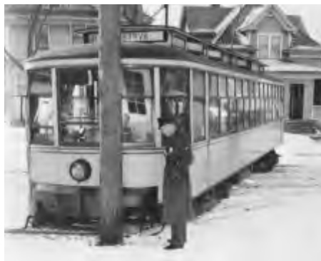
Oops. Patrolman Grant Williams studies the aftermath of this November 25, 1946 derailment on Rondo Avenue and St. Albans. Snow, or ice, compacted in the flangeway between the pavement and the rail caused a wheel to ride up and off the track. Rondo-Stryker would be abandoned and converted to buses two years later. St. Paul Dispatch and Pioneer Press photo, Minnesota Transportation Museum Collection.
