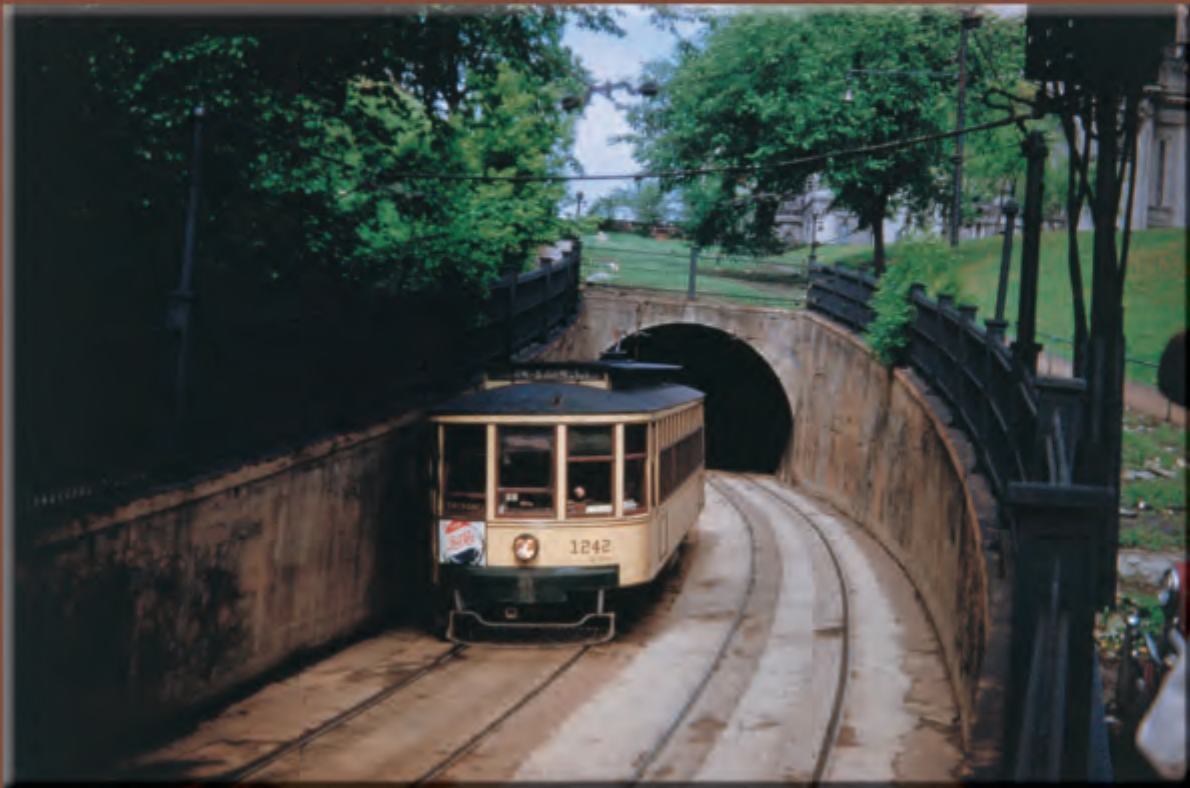
Selby Tunnel. A Selby-Lake car on its way downtown emerges from the east portal of the Selby Tunnel. Built to relieve the grade on Selby Hill and replace an awkward cable-counterweight system, the tunnel cost $366,000 when it opened in 1907. The west portal of the tunnel on Selby has been covered over and sealed. The east portal is still visible, albeit in considerably deteriorated condition. Minnesota Transportation Museum Collection.
