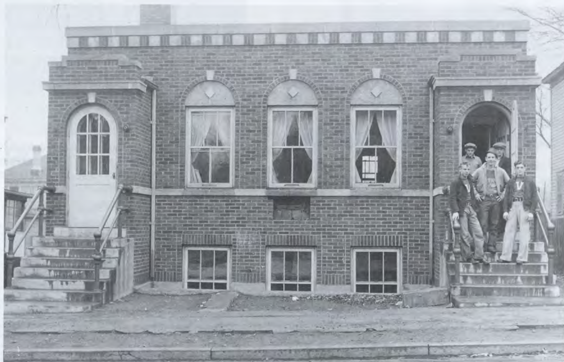
This is the Fourteenth Street Boys Club in 1933, which was formerly a mikvah. In ancient days, Jews used the mikvah as a place for ritual bathing. It was usually a body of natural water, such as a river or lake. Today a mikvah is located inside a building and looks like a small swimming pool that is filled with rainwater or water from a spring or stream. For many years, the residents of Fourteenth Street used a mikvah that was located on the old West Side flats, near the Mississippi River. In 1926 a group of wealthy Jewish men hired Max Buetow, a prominent architect, to design a mikvah for the property at 180 East Fourteenth, at the corner with Jackson Street. Using Buetow's plans, in 1926 they built this handsome, brick-and-tile,
