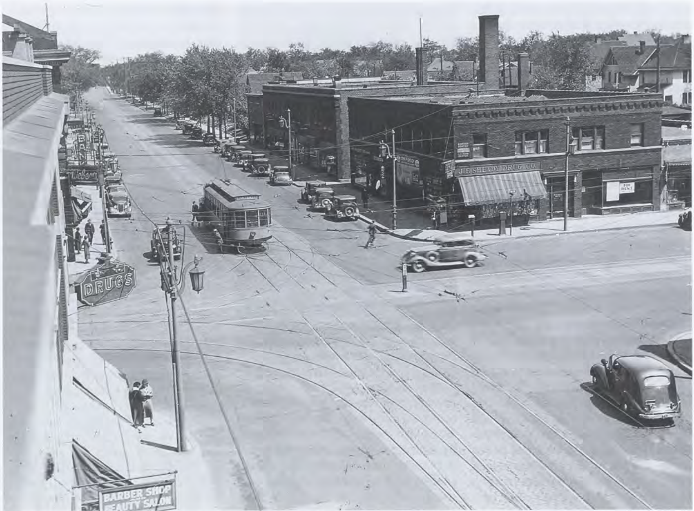
A photo taken from an elevated position looking east along Selby Avenue in about 1932 shows the intersection with Snelling Avenue in St Paul. The vertical post, near the center of the intersection and adjacent to the streetcar tracks, was a traffic control light. Sometime after this picture was taken, Park Drug and Park Liquor occupied the retail space shown in the top right-hand portion of the photo. Photo courtesy of the Minnesota Historical Society.
