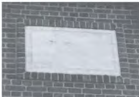
Detail, between windows, front of building, Arlington Hills Free Public Library, 1917. Photo courtesy of Lauren M. Freese.
