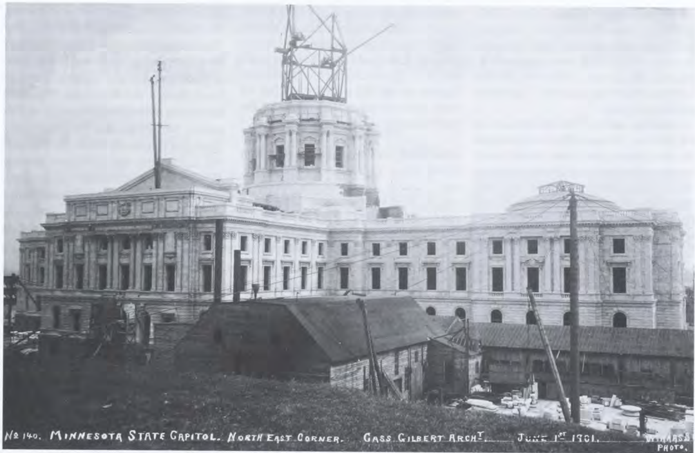
This 1901 photograph shows the Minnesota Capitol under construction. In the foreground is the stone cutting shed on the northeast side. The photo is from the collection of Channing Seabury, who was the chairman of the Capitol Commission, which oversaw the building's construction. Photo courtesy of Tom Blanck.
