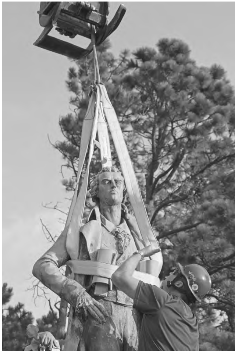
A crew from Saint Paul Parks and Recreation Department used a sling to carefully lift the statue from its granite pedestal prior to beginning the restoration work. Photo courtesy of Robert Muschewske.
