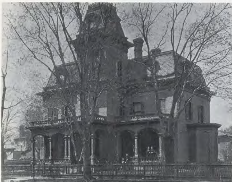
John S. Prince's massive Second Empire residence at 487 East Eighth street, about 1890. Minnesota Historical Society photo.
