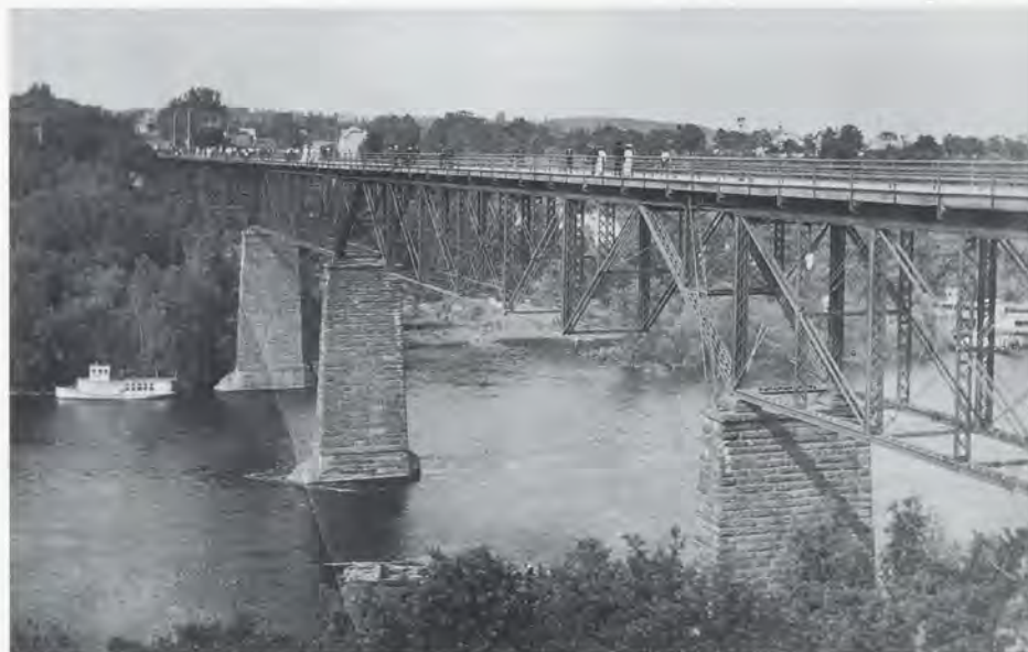
The Fort Snelling bridge in 1906, another example of a cantilever bridge. This view is looking toward the St. Paul side of the river. Minnesota Historical Society photo.
