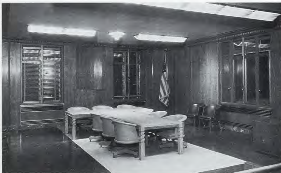
The county commissioners' board room as it looked about 1931, shortly after the new City Hall-County Courthouse opened. Photo from the St. Paul firm, formerly known as Ellerbe Associates, Inc., that worked with Holabird and Root of Chicago in designing the building.
