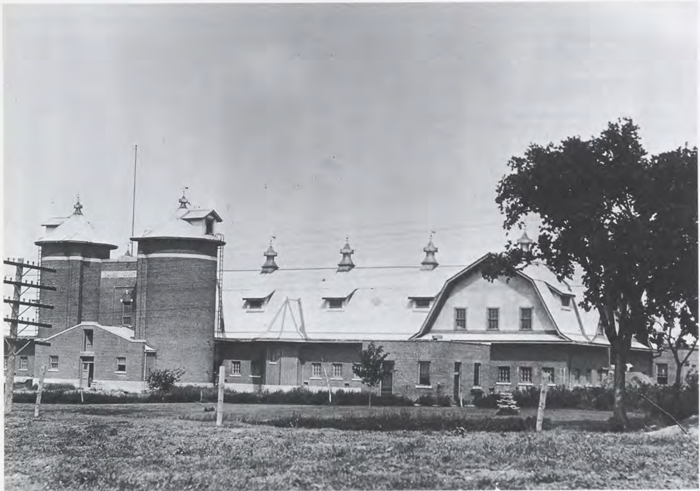
The cattle barn at the Ramsey County and a landmark since 1918. Now listed on the National Register of Historic Places, the barn, designed by St. Paul architects Buechner and Orth, replaced a frame structure built on the site in 1885. Cost for the pressed red brick structure was $56,198. Designed to hold seventy-five dairy cows, the barn is one of the largest of its kind in Ramsey County. Farming operations ceased in 1956 and the barn is now occupied by the Minnesota Extension Service. Minnesota Historical Society photograph.
