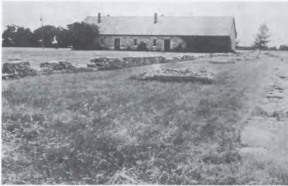
Foundations of the buildings at Fort Ridgely as they looked in this 1959 National Park Service photograph.
