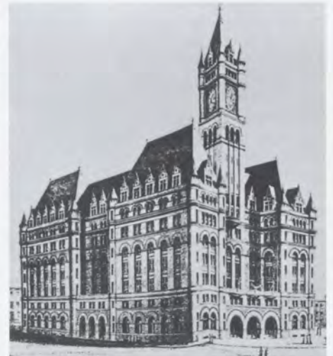
Another building bearing a strong resemblance to the Old Federal Courts Building and built about the same time: the United States Post Office in Washington D. C. This design appeared in the American Architect and Building Review for March 12, 1892. Photo from the Minnesota Historical Society.
