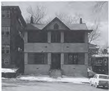
Before restoration: the house J. Jay Knox and his brother Henry built in 1860. After 1910, the house was covered with stucco. Photos are from the Minnesota Historical Society and the Ramsey County Historical Society.
