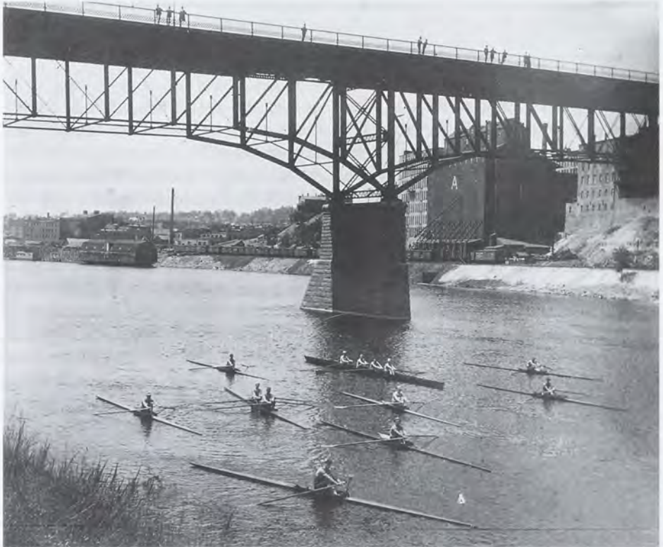
A race circa 1895 on the Mississippi River below the Wabasha Street bridge, which had been rebuilt, its old wooden trusses replaced by wrought iron.
