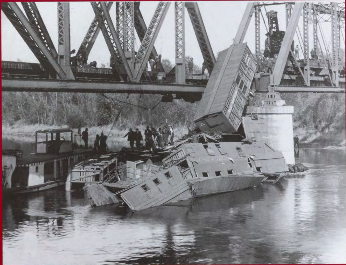
The wreck of Terminal Railway's No. 10 on October 15, 1912 when the 145,000-pound locomotive, tender, and eight cars plunged off the railroad's swing bridge into the Mississippi twenty-five feet below. Photograph from the Davis, Kellogg and Severance Case Files at the Minnesota Historical Society collections. See article beginning on page 4.
